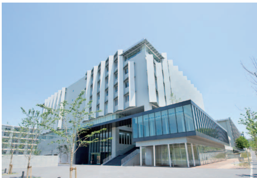
ES 総合館 Engineering and Science Building
