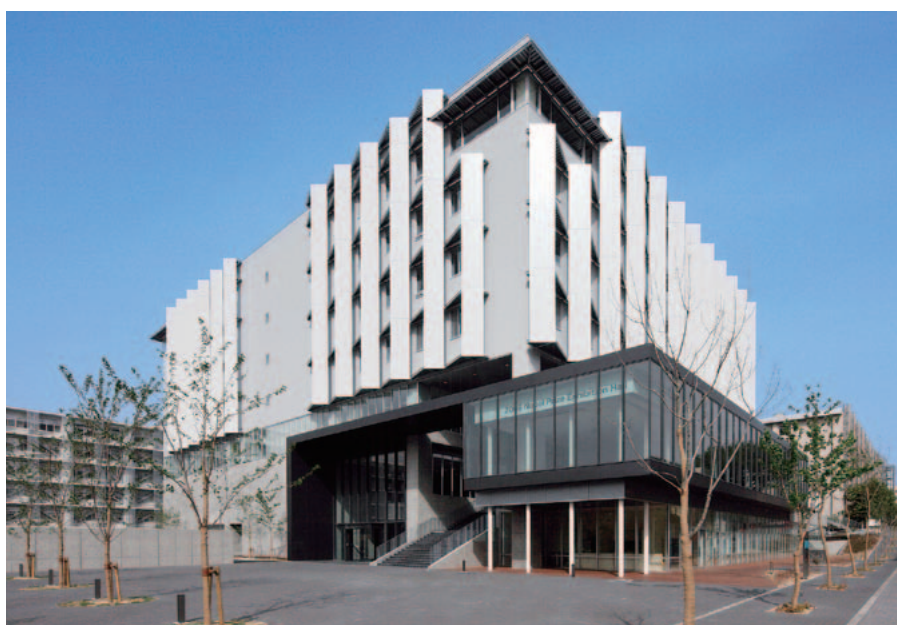
ES 総合館 Engineering and Science Building
